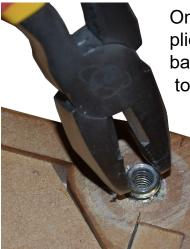
Once the glue had set, I used pliers to screw the insert nut back into the cavity. Thanks
