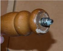
in place. The insert nut was no longer anchored in place, so the leg just dropped out. When I unscrewed the leg, the nut came out right along with it.
